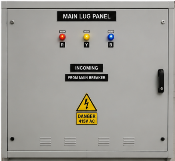
MAIN LUG PANEL – FRONT VIEW
