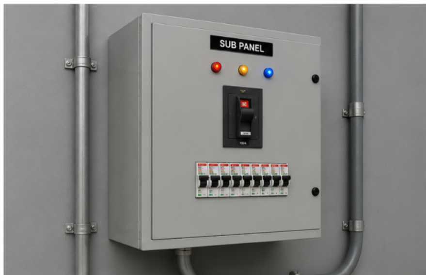
4. SUB PANEL – SURFACE MOUNTED VIEW
